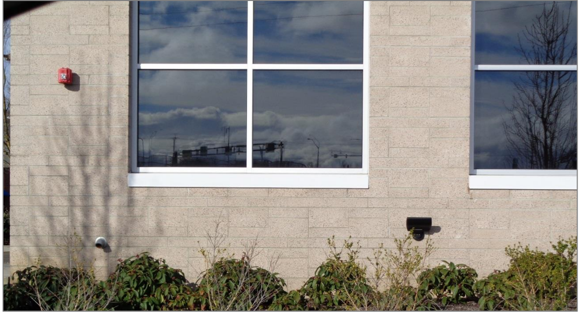
CMU wall (Red Robin, 3060 Sprague Ln, view along Arney Rd)
