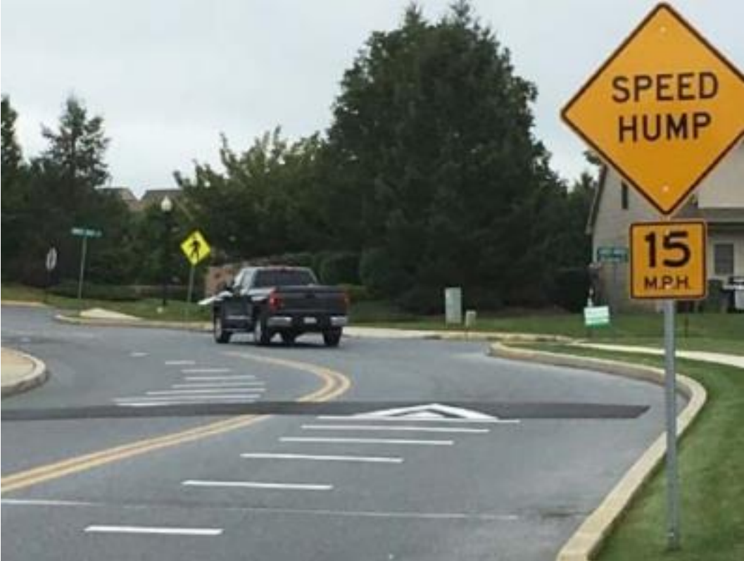
Figure 2. Example of a Speed Hump. Source: ITE Traffic Calming Fact Sheets.
