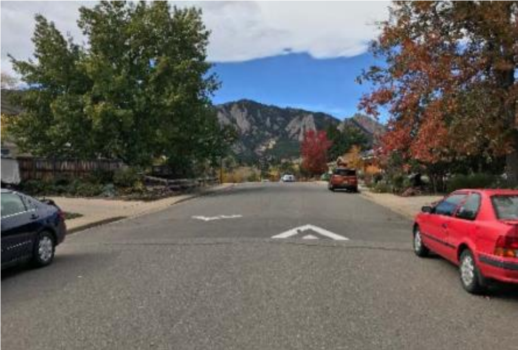
Figure 1. Example of a Speed Hump. Source: ITE Traffic Calming Fact Sheets.
