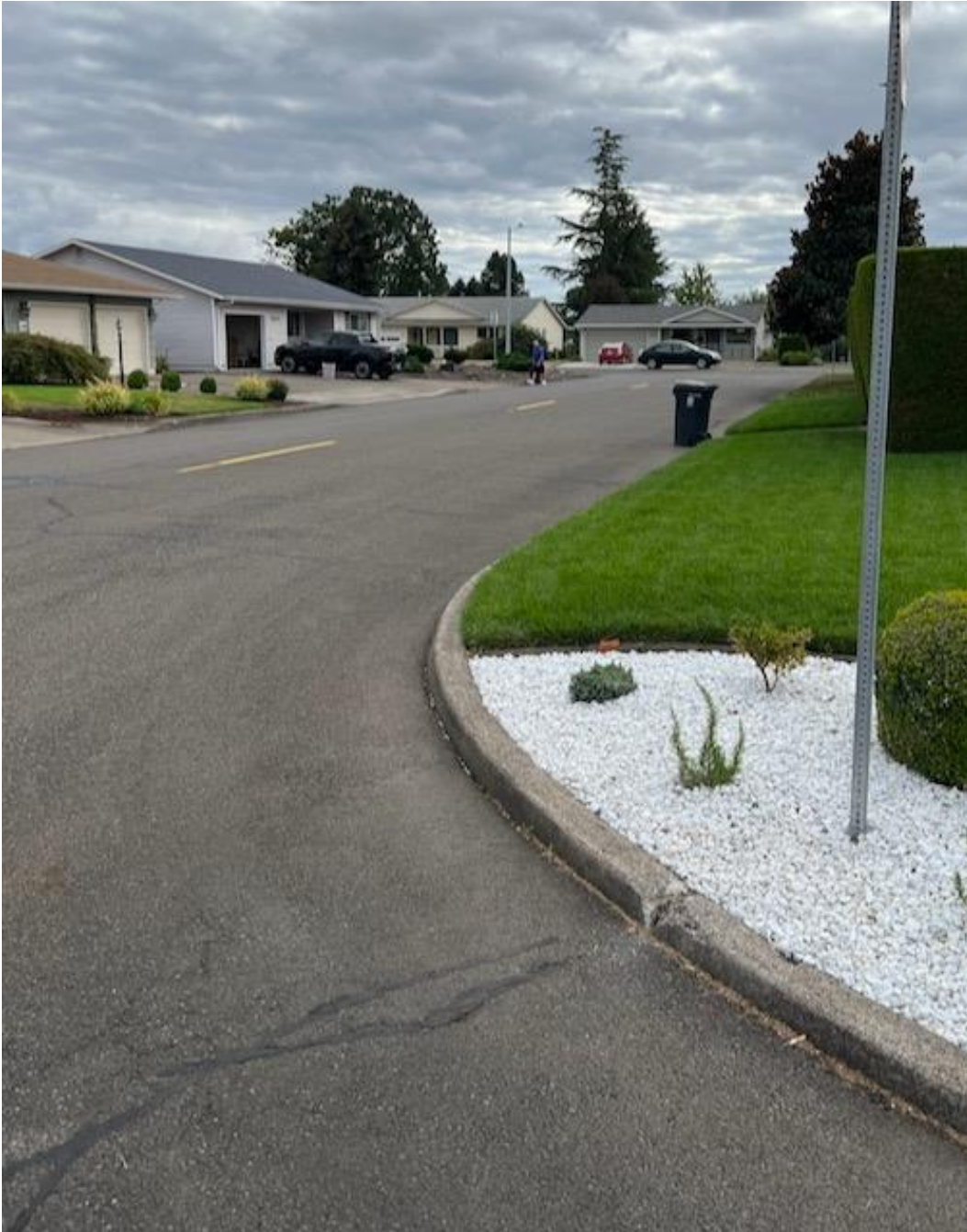
Figure 5. View from Oregon Court facing south.
