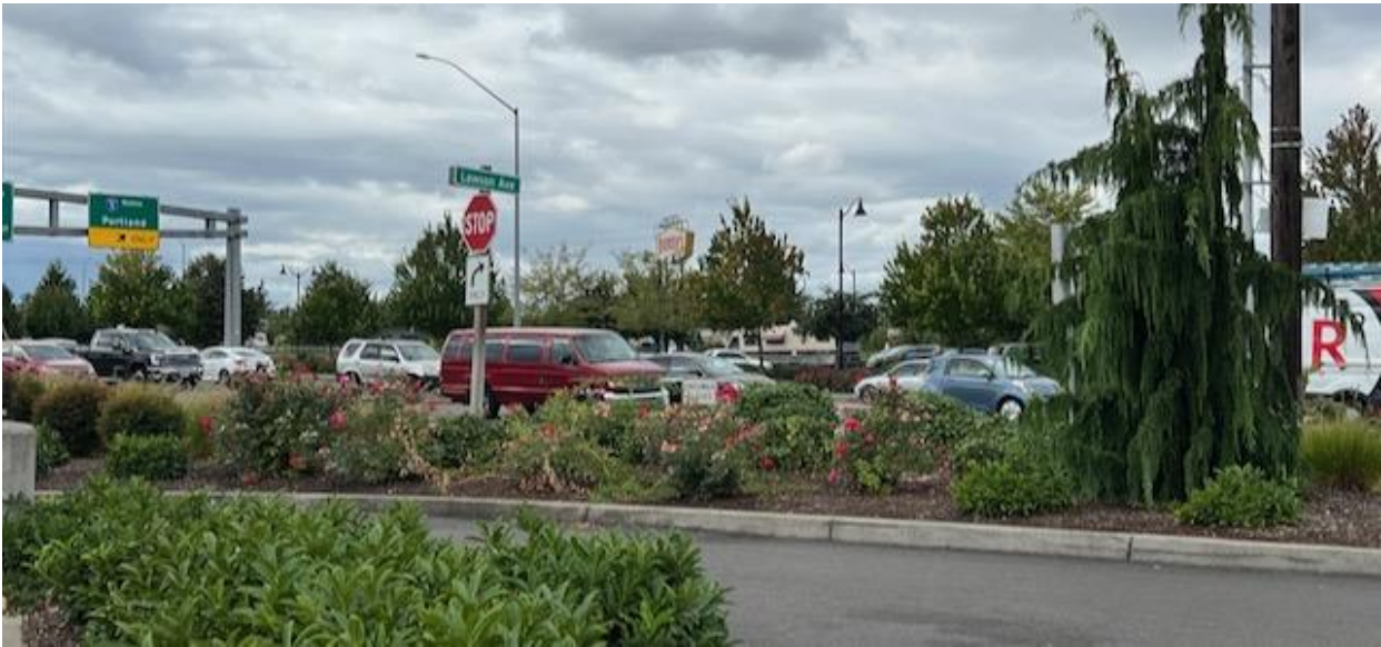
Figure 16. View from the southeast quadrant of OR 214/Lawson Avenue toward I-5 showing that eastbound OR 214 queues commonly extend beyond Lawson Avenue.
