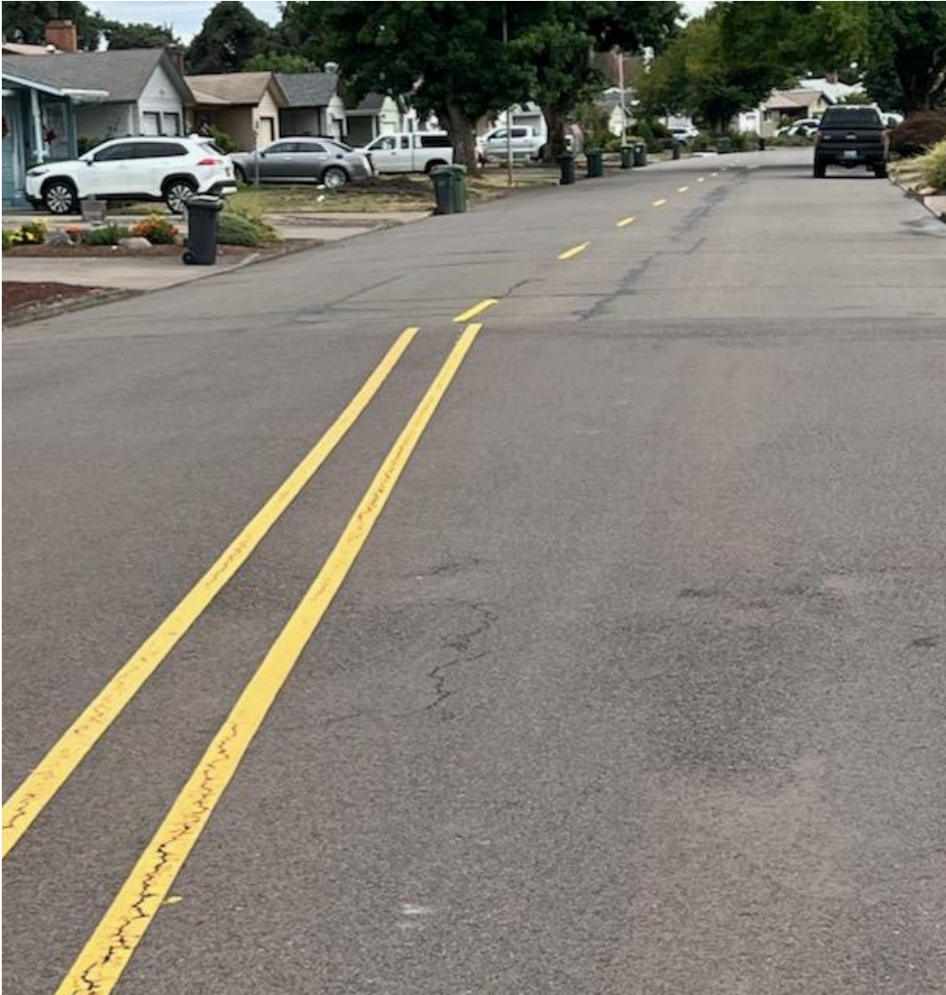
Figure 3. Existing skip striping along Oregon Way.
