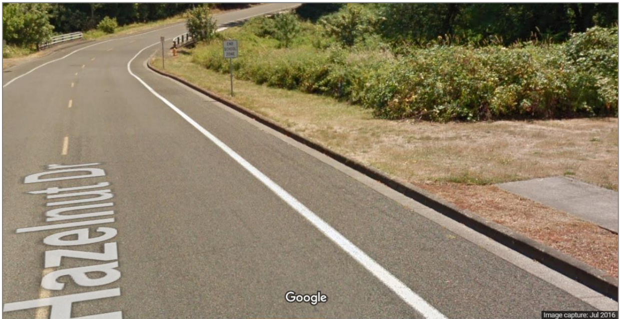
Google Street View (2016) east along Hazelnut Drive of sidewalk gap up to Mill Creek culvert crossing sidewalk
