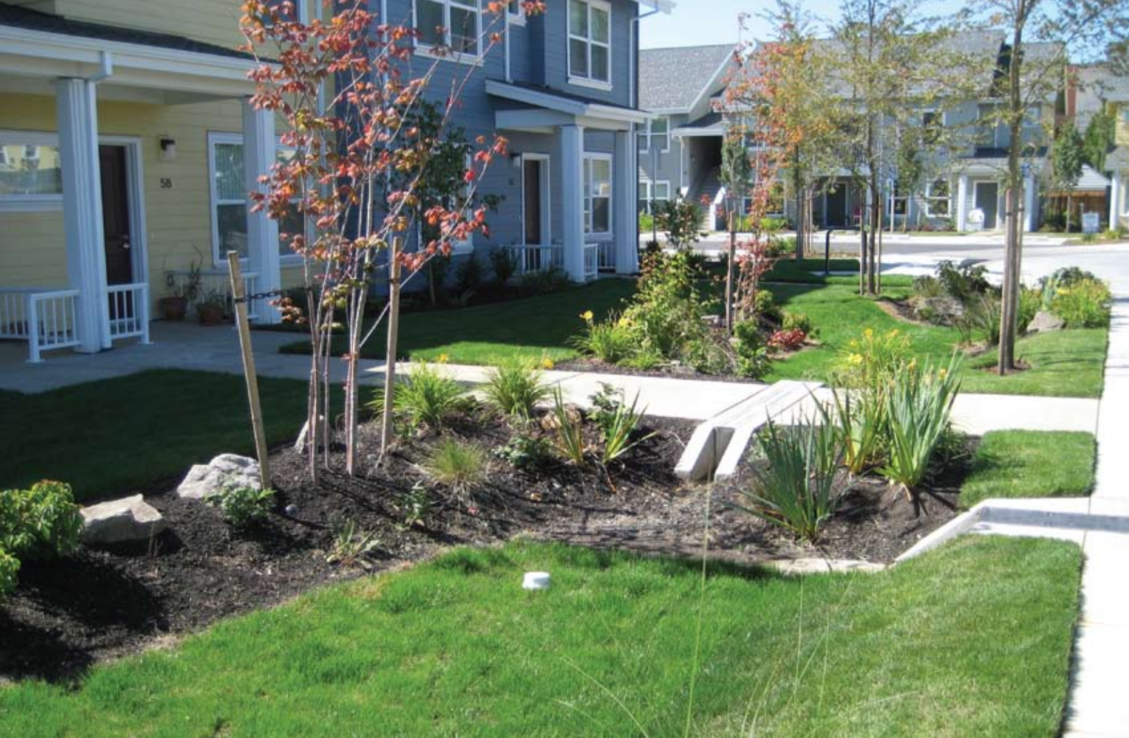
Figure 34: Rain garden using a grassy swale as the base. (Photo: Candace Stoughton, EMSWCD.)
