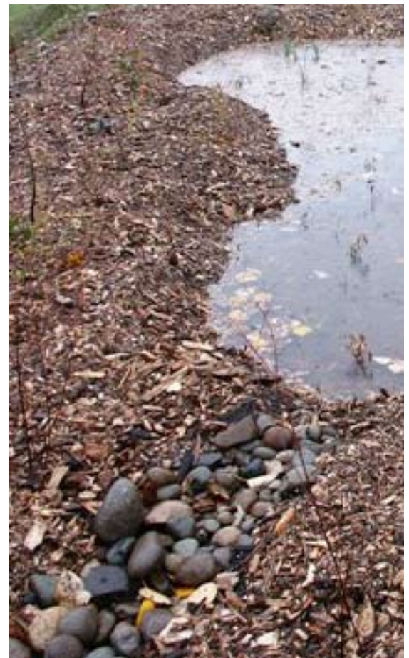
Figure 17: Outflow notch in a Washington rain garden. (Photo: Curtis Hinman, WSU)
