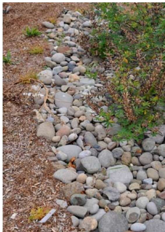
Figure 11: Using a rock-lined trench to convey water across a walkway (Photo: Portland Bureau of Environmental Services [BES])
