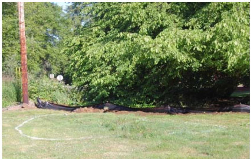
Figures 9a and b: Delineating rain garden boundaries with a garden hose (top) and marking paint (above). (Photos by Robert Emanuel, OSU)
