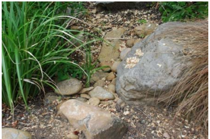
Figure 24: Rock, gravel, and sedges protect the inflow point in a coastal rain garden. (Photo: Robert Emanuel, OSU)
