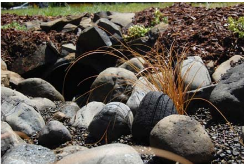
Figure 25: An outflow notch in a Portland, Oregon, rain garden, protected by rock to prevent soil erosion. (Photo: Chris LaBelle, OSU)
