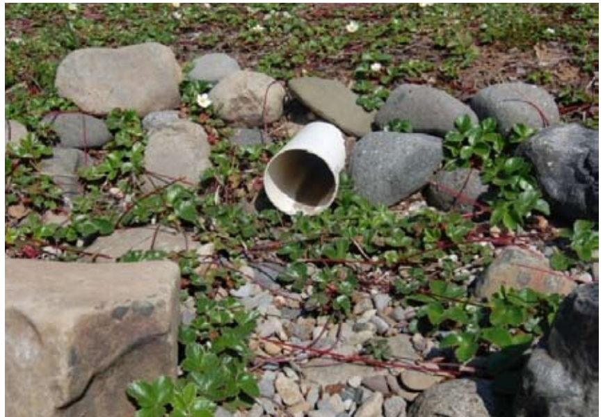
Figure 23: The point where water enters a rain garden should be well armored with rock and plants (beach strawberries here) to prevent erosion. (Photo: Robert Emanuel, OSU)
