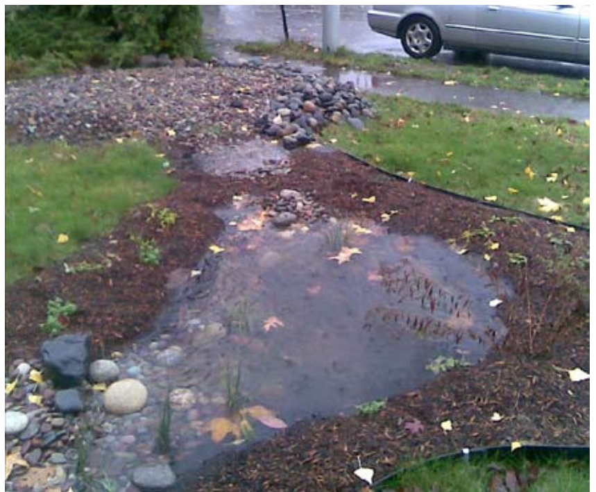
Figure 31 (right): A rain garden in Gresham, Oregon fills with rain. Note the use of rocks at inflow and outflow points to minimize erosion. (Photo: City of Gresham)
