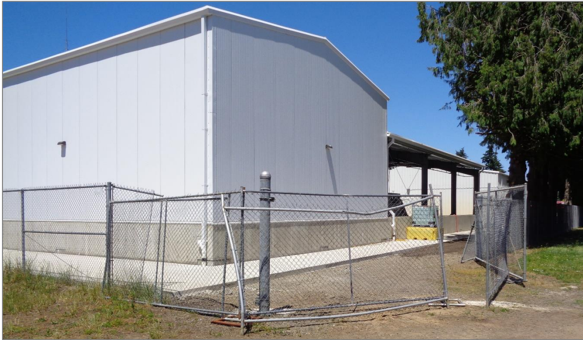
Site southeast corner, June 12, 2024
