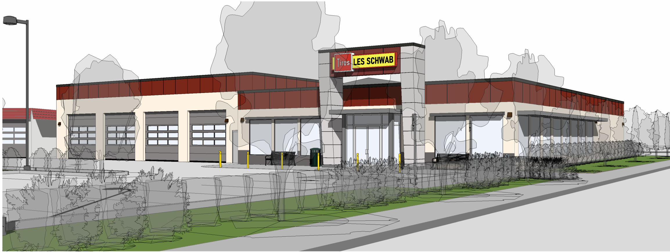
NORTHWEST VIEW FROM N PACIFIC HWY
