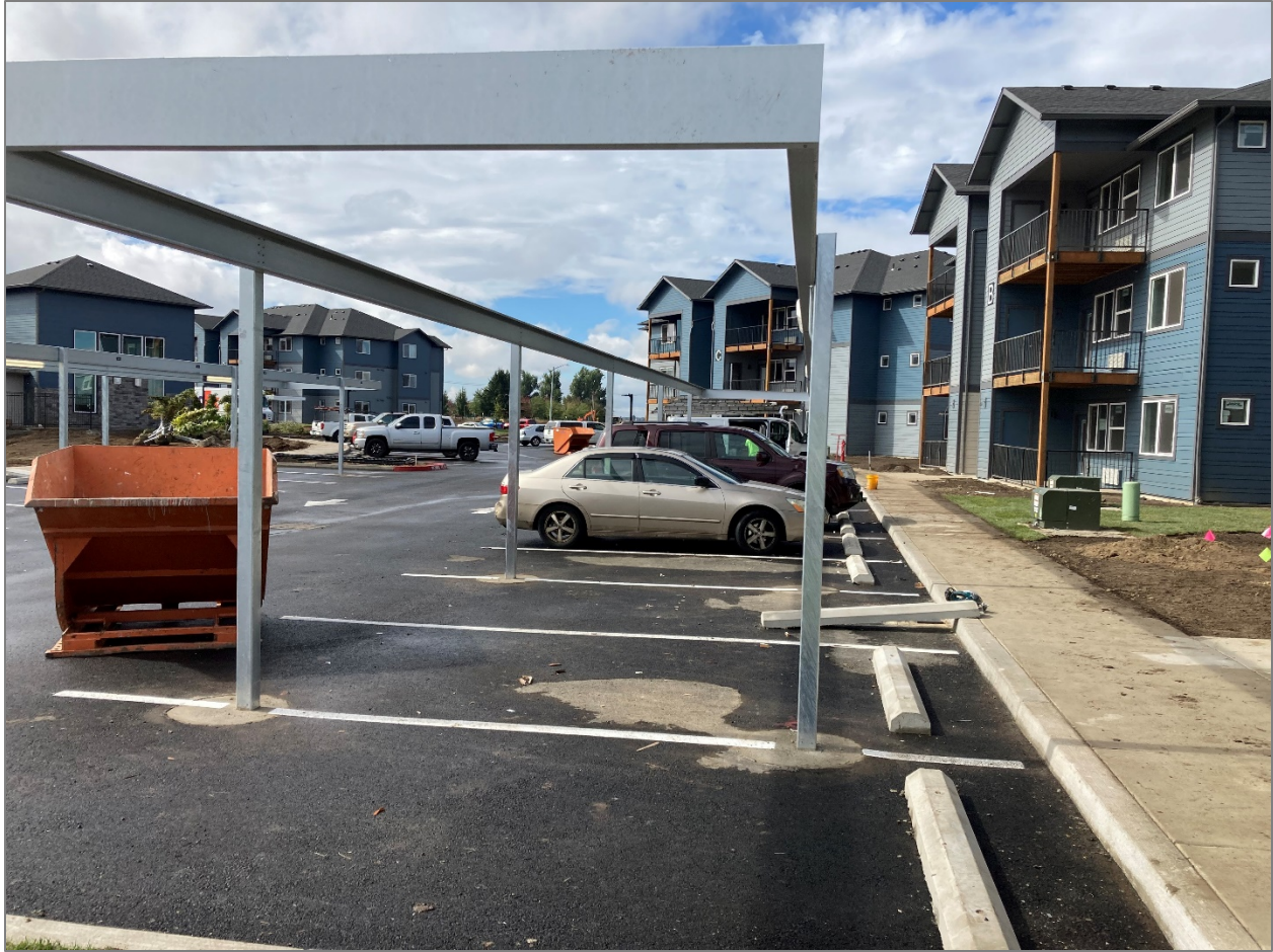
Carports at Smith Creek Apartments (site inspection on 9/28/2022)
