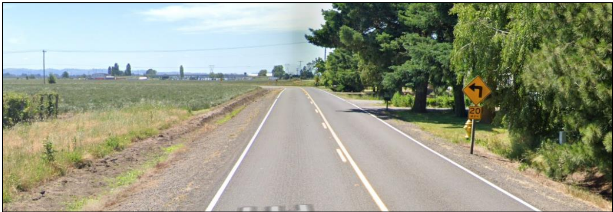
Figure 3: Parr Road Looking West at 90-Degree Curve (© Google Street View, June 2019)
