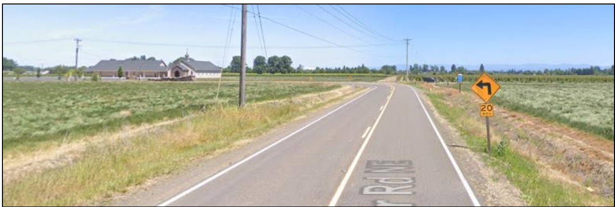
Figure 5: Parr Road Looking East at 90-Degree Curve to North (© Google Street View, June 2019)
