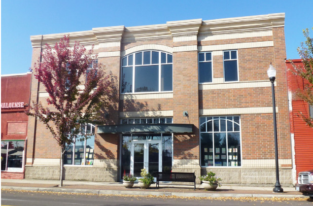
Front Street Façade
