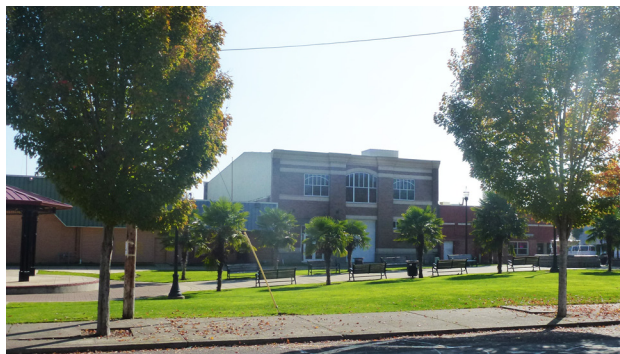
Association Building's location on the Downtown Plaza and alley
